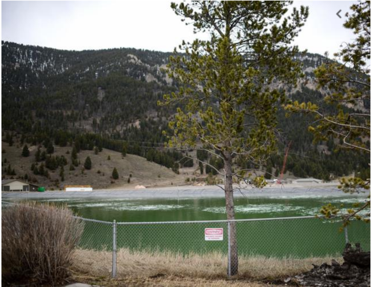
Pine trees grow inside a chain link fence surrounding the sewage and water holding ponds at the Big Sky County Water & Sewer Rachel Leathe/Chronicle
